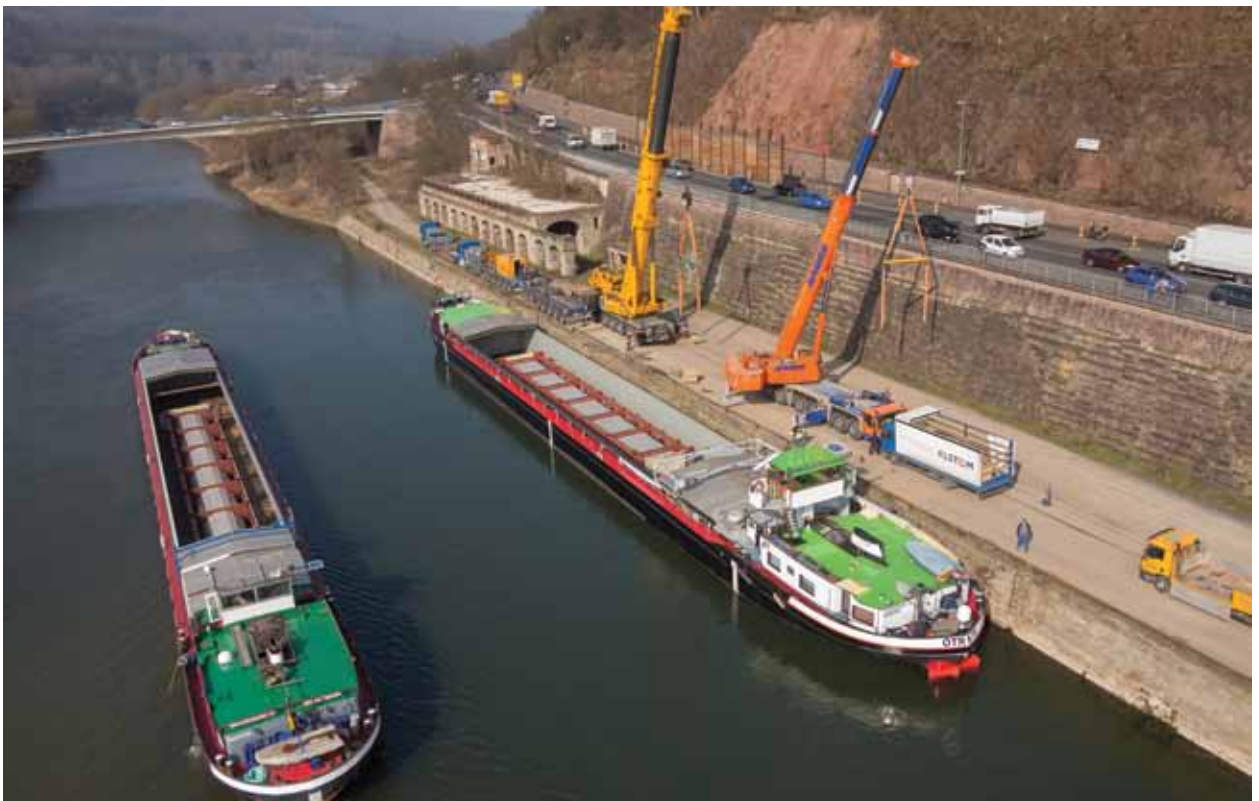
Handling of an abnormal load at the Weser transshipment facility Hann. Münden
