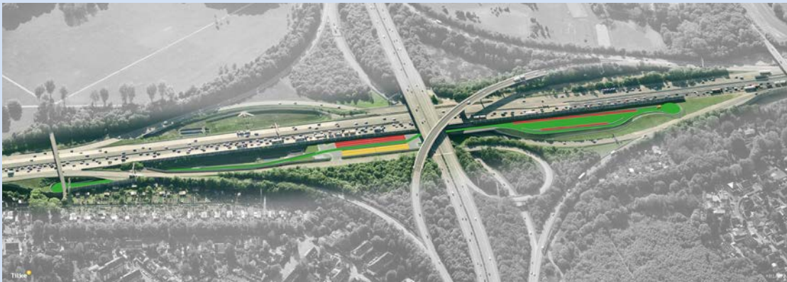
Demonstration and test site (duraBAST) © Tilke/BAST
