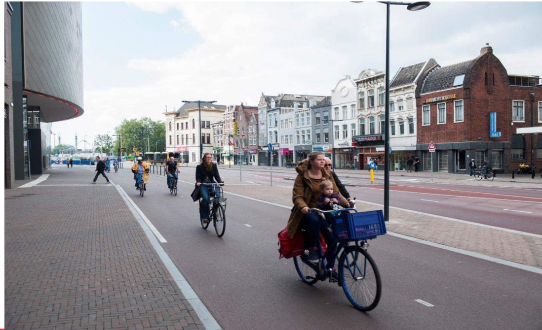
Utrecht Two-way cycle track dedicated to the busiest traffic corridor: 25.000 cyclists per 24 hours
