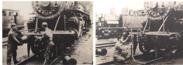
Fig. 3: Conversion of a Japanese locomotive from SC to “Janney” AC
